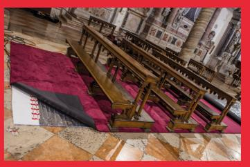
This heating system is completely invisible and silent and in no way disturbs the sight and hearing.
