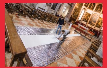
The Warmset underfloor heating system can be laid without any masonry work.
