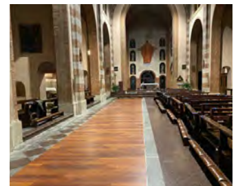
Laying of flooring and closing profiles
