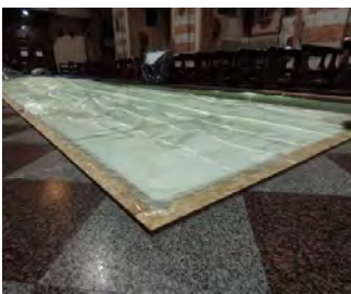
Laying of styrodur insulation and chipboard frame
