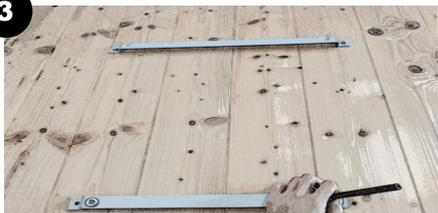
Therefore also fix the bracket **B** (with magnet) to the wall. This bracket will be used to leave the panel not in direct contact with the wall and to stabilize it.
